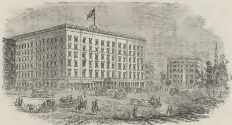
FIFTH AVENUE HOTEL. FIFTH AVENUE AND BROADWAY.
